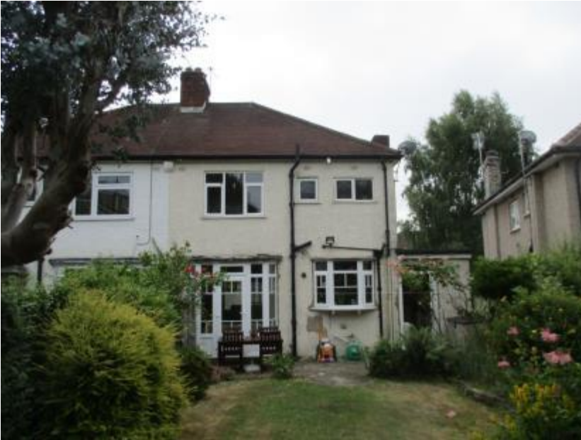
Rear of 53 – no. 51 to the right
